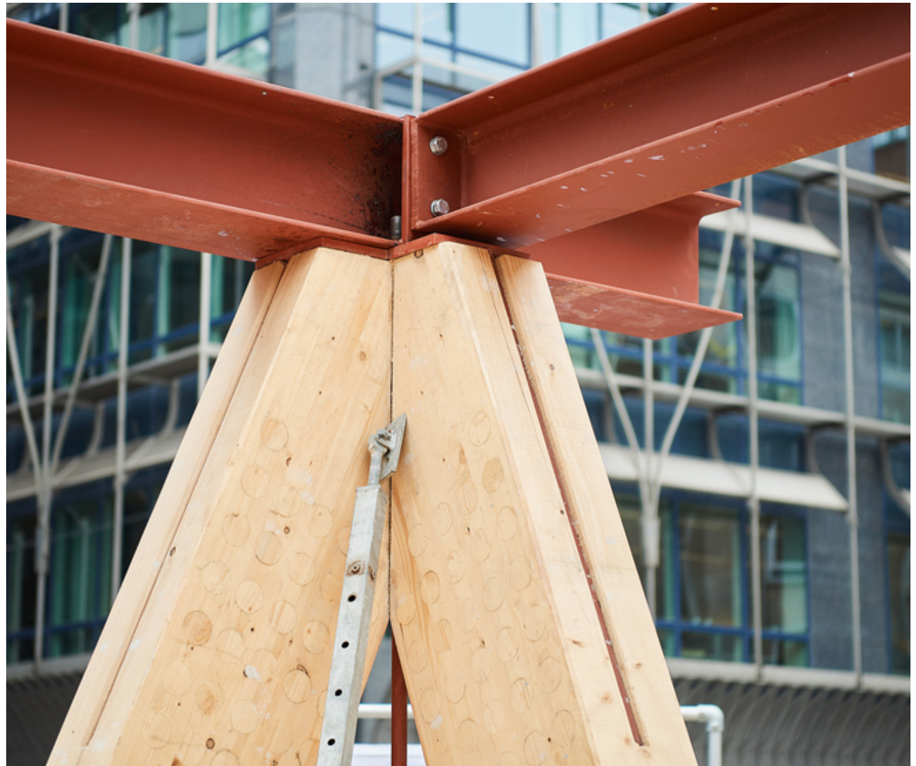
► Detail of the innovative timber structure of the office building Montoyer 10 (M10) – Brussels's CBD (BE)
