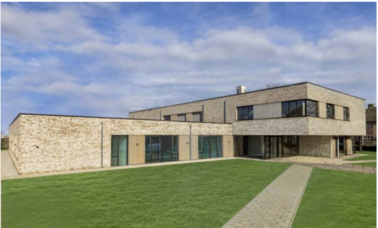
► Medical office building - Sittard (NL)
