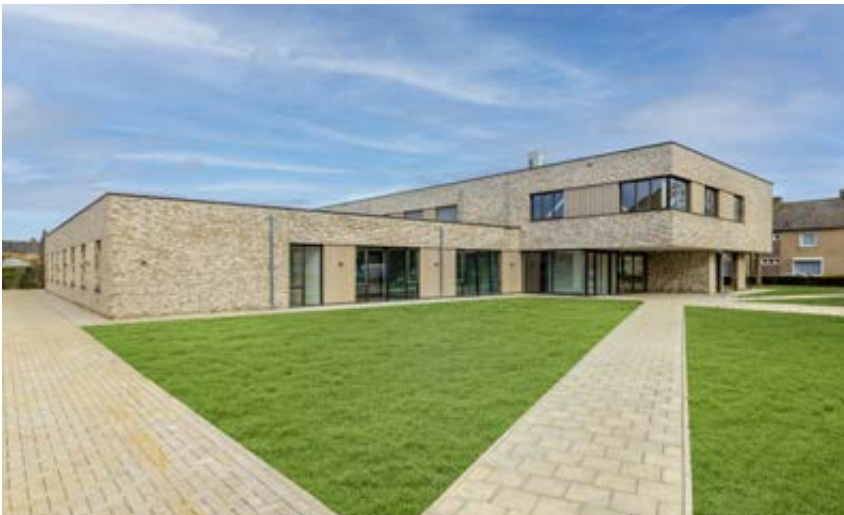
► Medical office building - Sittard (NL)
