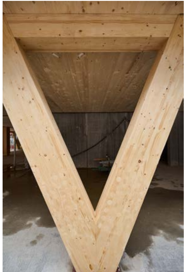
► Detail of the innovative timber structure of the office building Montoyer 10 - Brussels' CBD (BE)
