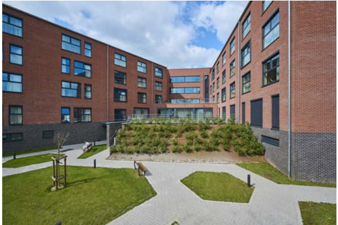
► Nursing and care home Clos de la Rivelaïne - Charleroi (BE)
