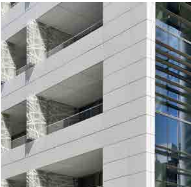
► Office building Belliard 40 - Brussels CBD (BE)
