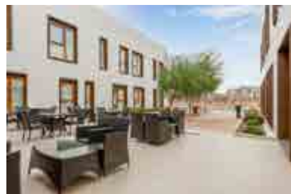
► Nursing and care home - Castellón de la Plana (ES)
