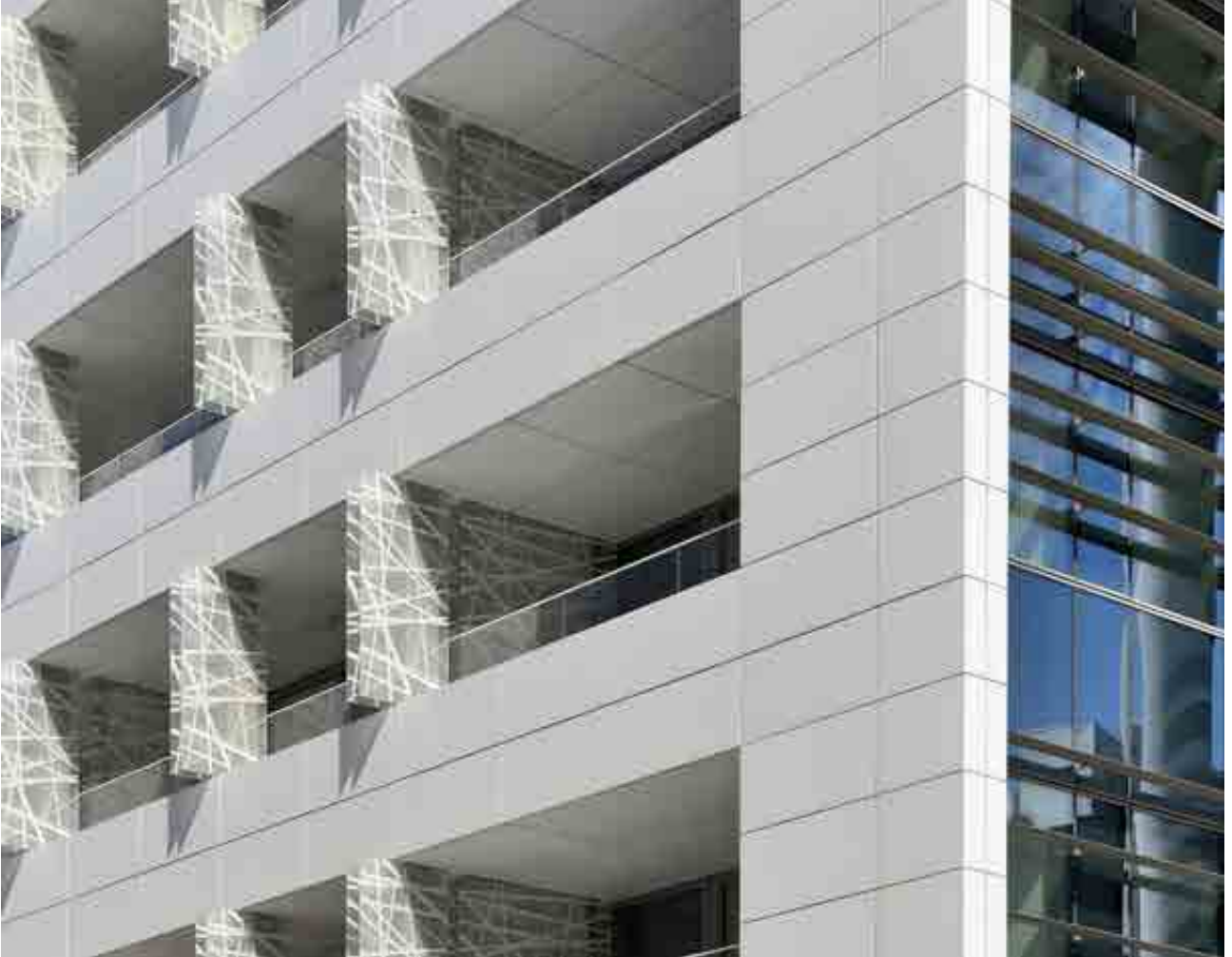
► Office building Belliard 40 - Brussels CBD (BE)
